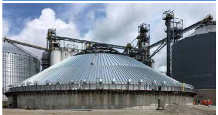
First Behlen two million bushel bin under construction in Ohio.
